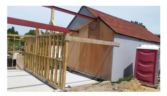
29. The left of this photograph shows the western end of the building, with new floor, foundations, stud work and supporting steels apparent. This is plainly not a conversion. On the other hand, the right hand side of this photograph shows the eastern end, which includes the original roof of the building, including internal structural elements, as the following picture shows.
